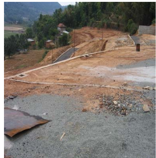
Photo of unapproved site
